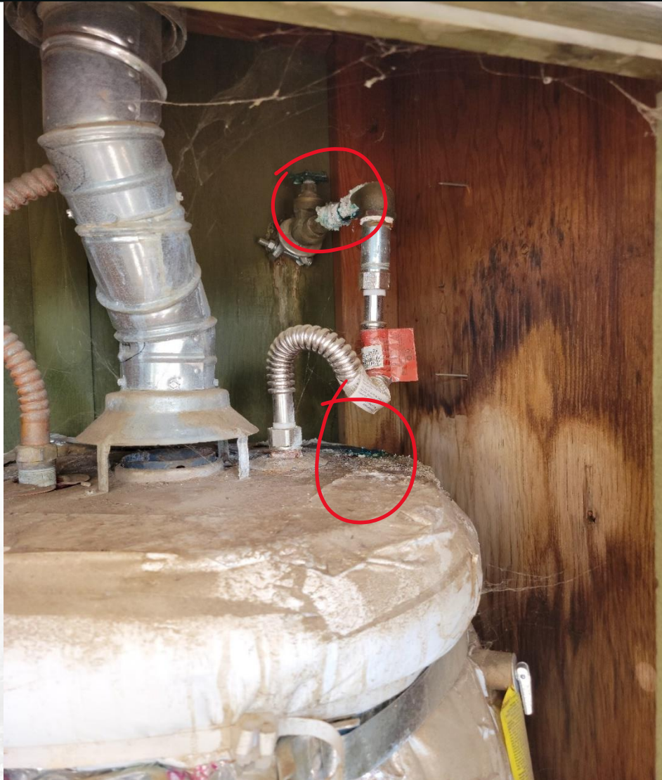
Leak and Corrosion
