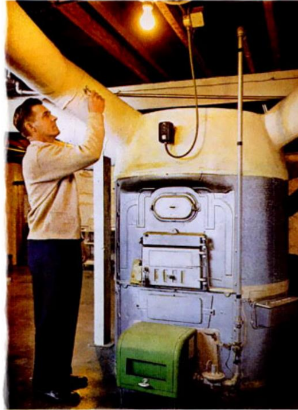
"Before we switched to electric heat, this monster took up a lot of living space."
