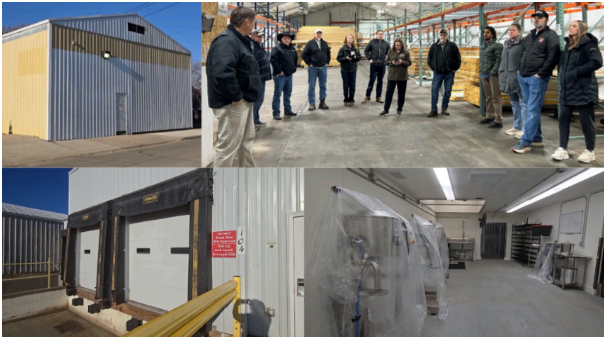
Photos: Interior and exterior of the Velva facility, top right photo shows stakeholders touring the facility
